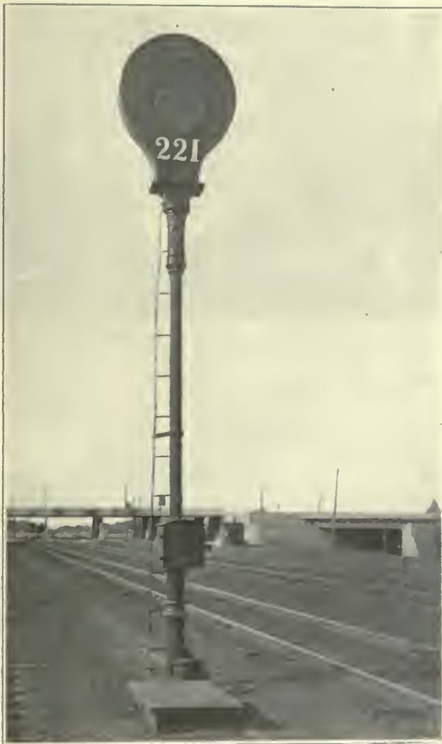
FIG. 282. SIGNALS. Disc signal ("Banjo" type) on the Illinois Central Railroad near 76th Street.
